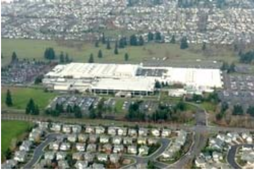
An aerial view looking north at Hewlett-Packard on SE 34th St. east of 164th Ave. (File/The Columbian)
